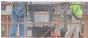
Workers using harnesses and lanyards
